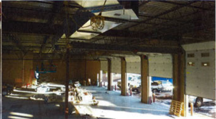
Shop Garage Door installation
